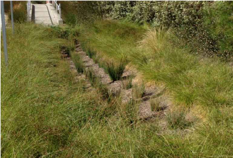
Bioretention basins throughout Verano Place Unit 6 apartments filter storm water through a soil medium and through phytoremediation.
