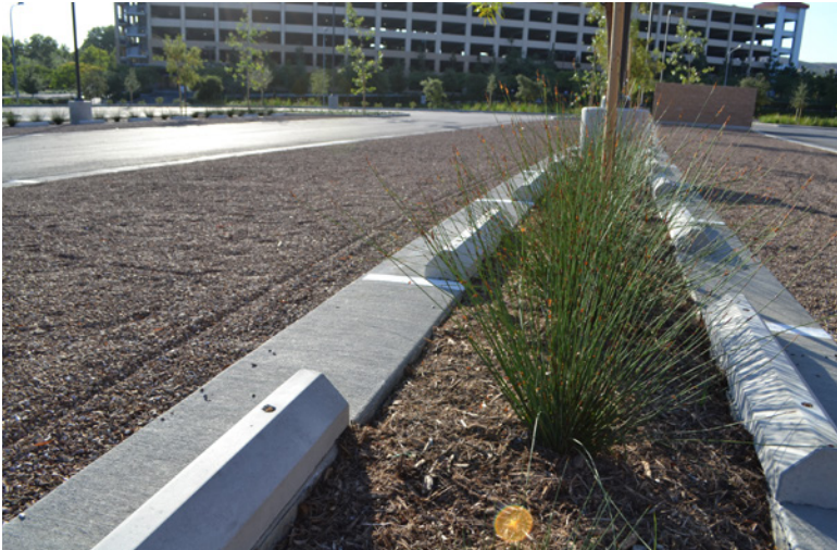
The parking lot at Verano Place Unit 6 graduate student apartments used permeable pavement as part of earning four LEED Platinum certifications from the U.S. Green Building Council (USGBC).
